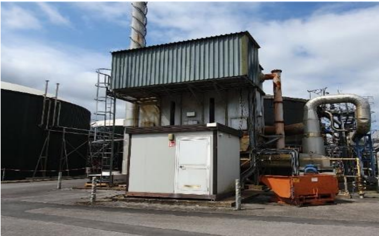
FIGURE 6-13: EXISTING RTO TO BE DEMOLISHED
