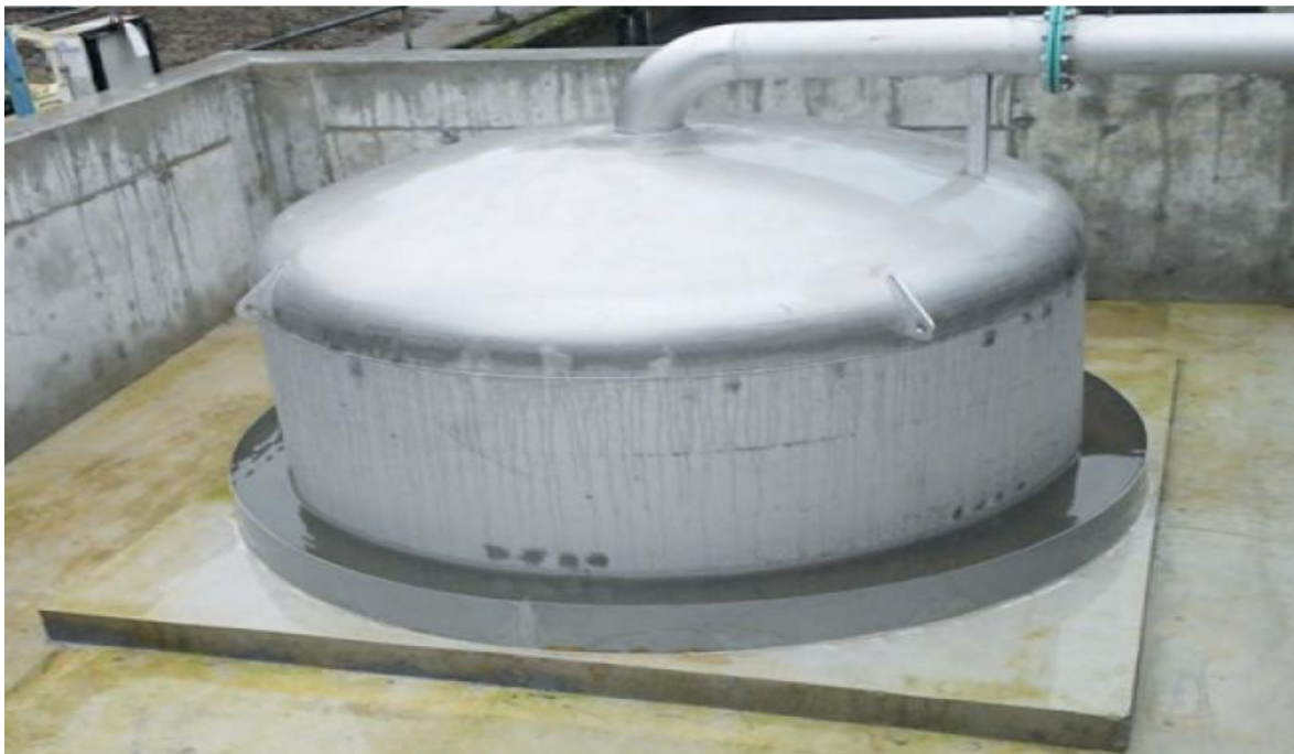
FIGURE 6-10: EXAMPLE OF FLUSHING BELL SYSTEM
